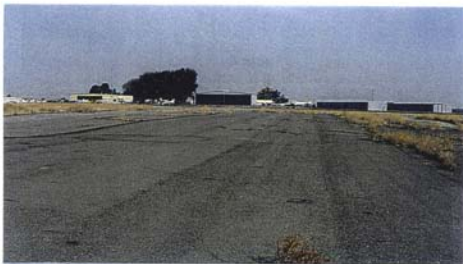
TERMINAL AREA FROM THE SOUTH LOOKING ACROSS THE RUNWAY
